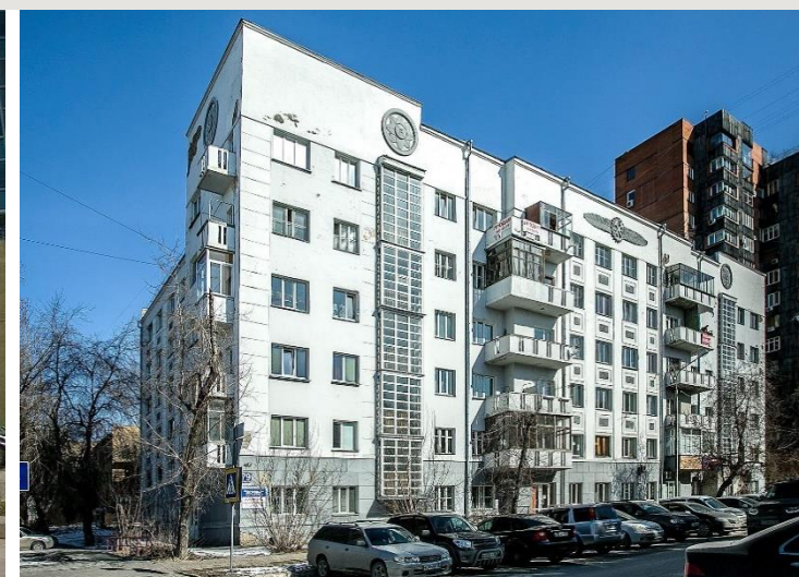
Residential building "Sibzoloto" (Soyuzzoloto)
